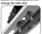
**4.** Tighten down to specified torque rating of 8Nm.
